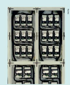
The 8562 series of flameproof MCBs is arranged and wired in 8125 enclosures. The enclosures are connected to each other by flanges. The feed is supplied through a busbar system, and the outgoing leads are collected together in terminal blocks.
