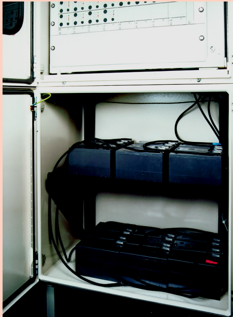
The batteries are installed in the battery cabinet
