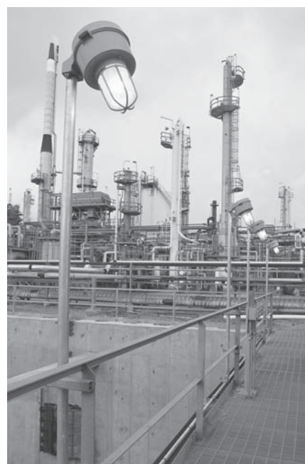
Enclosed and gasketed CHAMP ® luminaires providing walkway lighting
