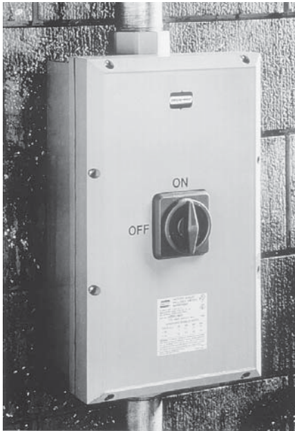
N2RS Factory-sealed industrial control switch
