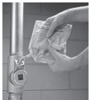
CHICO A-P INTRAPAK® premeasured sealing compound and water in plastic mixing pouch
