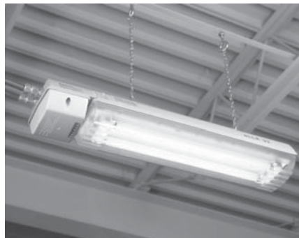
SpecOne™ eLLK Luminaire is CUL certified for Class II, Division 1 locations.
