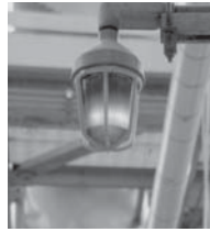
VAPORGARD™ luminaires in oil refinery
