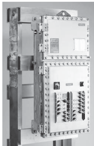
D2LU Lighting Panelboard Rack Mounted
