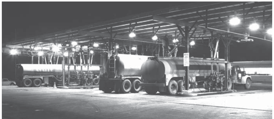
Tank truck loading platform
