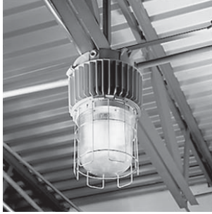
This CHAMP® DMV luminaire with guard provides aisle lighting in a storage facility.
