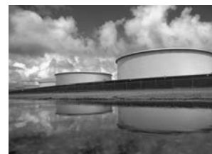
Waste Water Treatment
